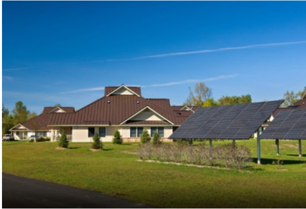
Quad-plexes and PV arrays Photo: Akwesasne Housing Authority
