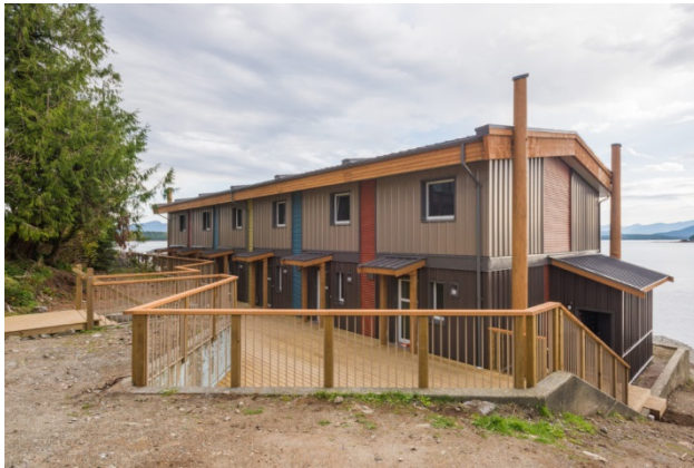
Stacked modules form the six staff housing units Photo Credit: Mobius Architecture
