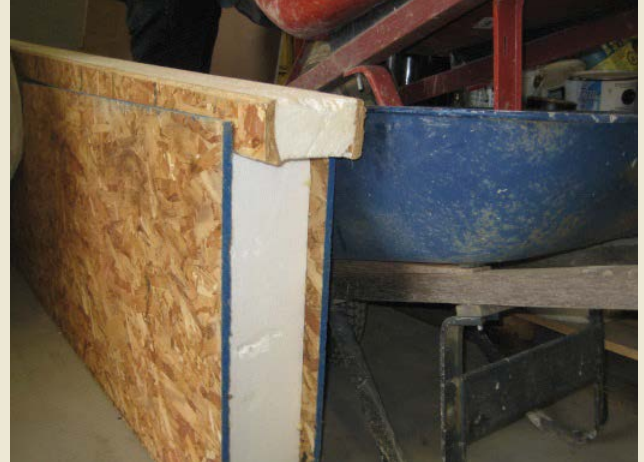
Figure 1 Structural insulated panel
