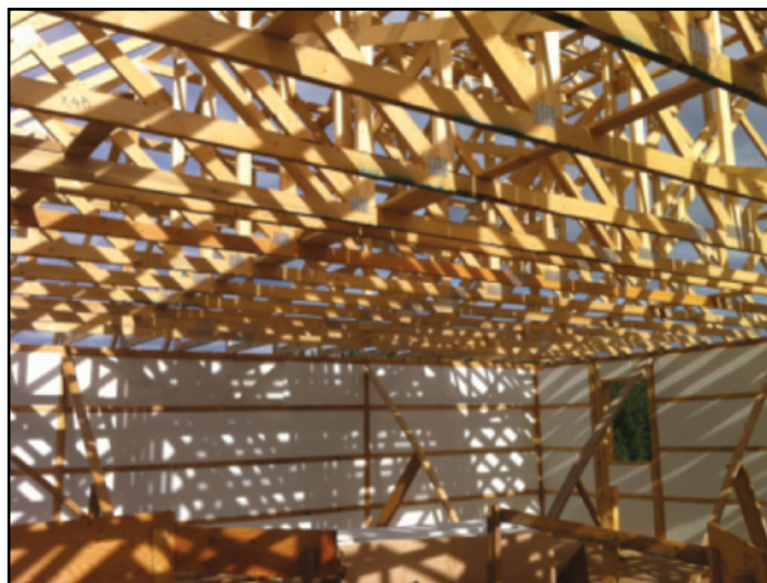
Figure 4 Roof framing
