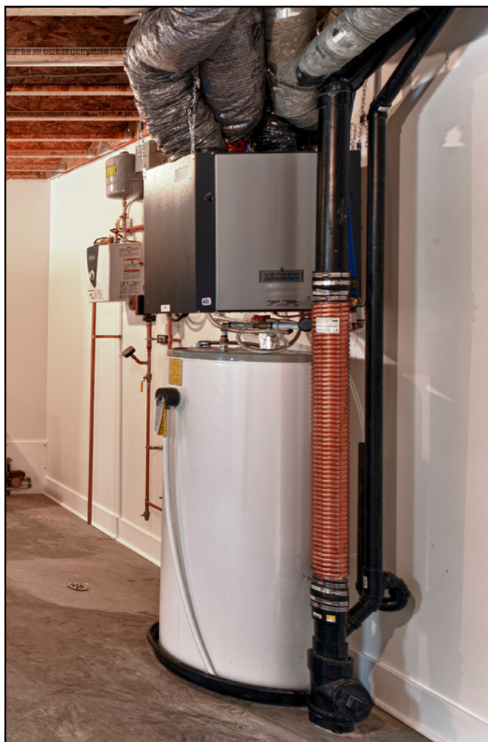
Figure 5 Heat recovery ventilator (HRV), hot water and drainwater heat recovery system
