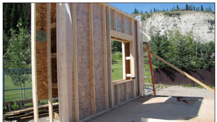
Figure 3 Larsen truss wall system construction
