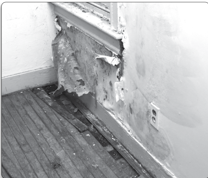
Water damage under a window
