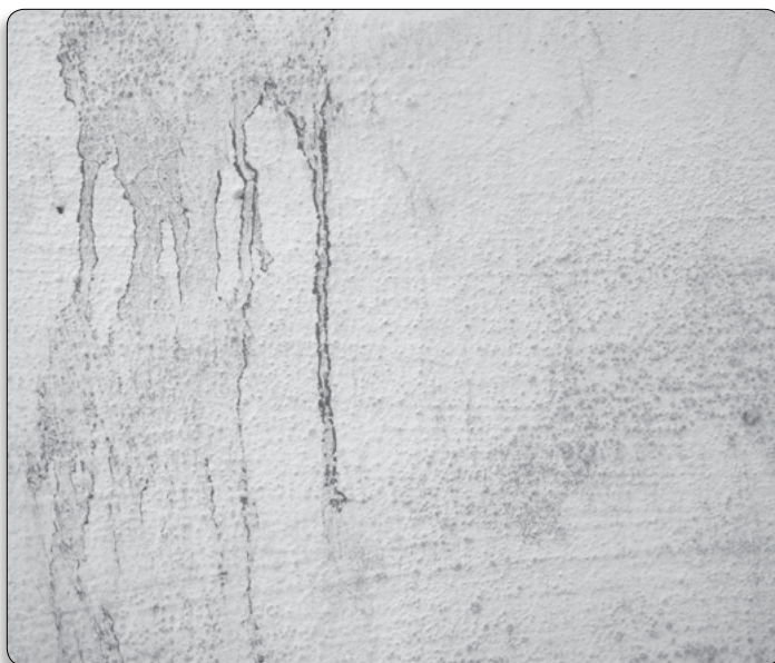
Stains on materials often indicate water damage
