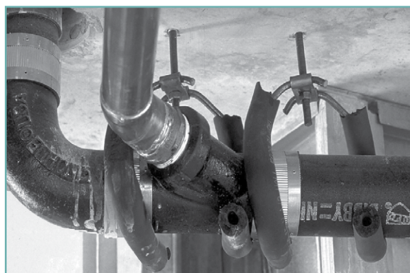
Figure 4-14 Plumbing penetrations
