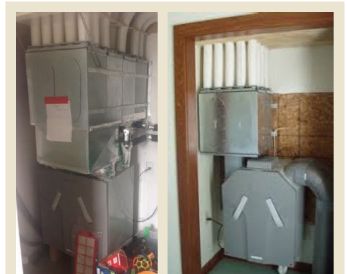
Figure 4.5 Examples of in-suite HRV units serving multiple zones. The unit on the left is actually serving an extended family home, so it has many more duct connections (one per room) than a typical MURB suite would have. The size of the unit is comparable to what would be used in a suite (images courtesy of Bernhardt Contracting Ltd.).
