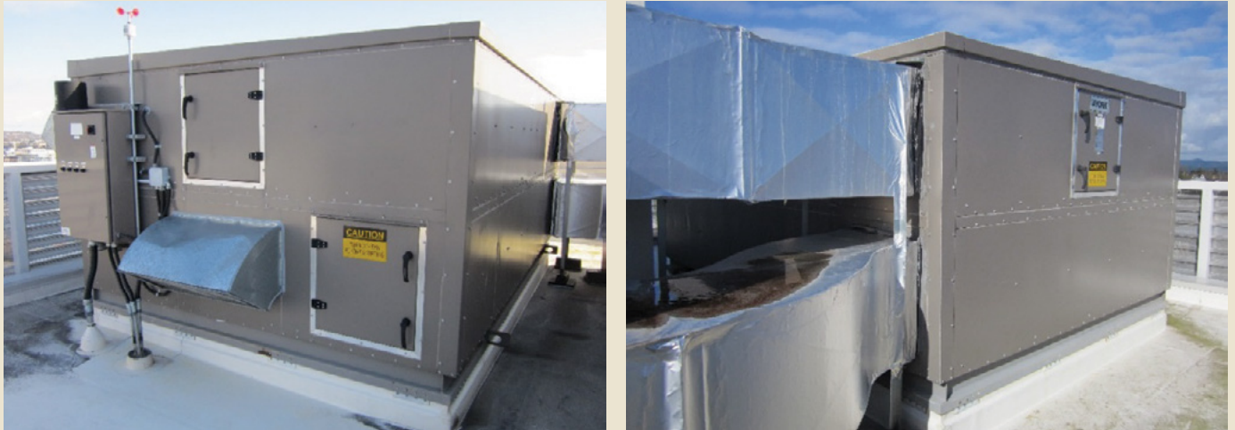
Figure 4.4 Custom centralized HRV for an 11-storey MURB. The unit supplies ~6000 cfm to 90 units.
