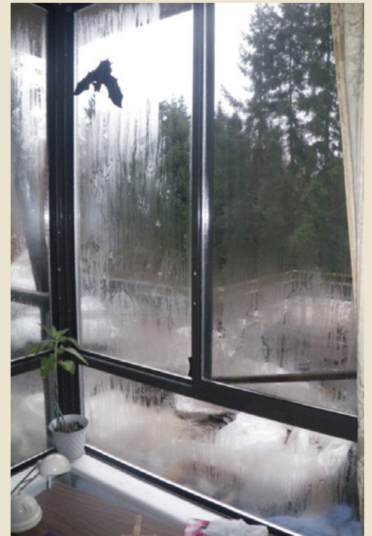
Figure 1.2 Condensation on the interior surface of windows
