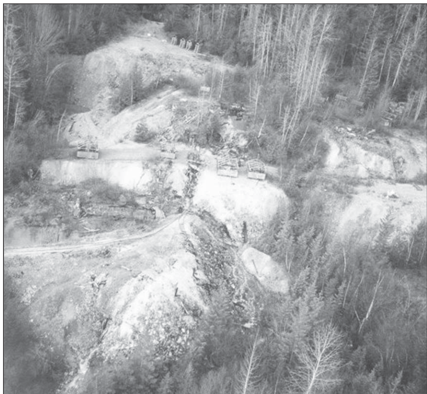
Partially reclaimed abandoned mine from the 1950's. Acid mine drainage is an ongoing closure issue at this site. Photo courtesy of TRTFN.
