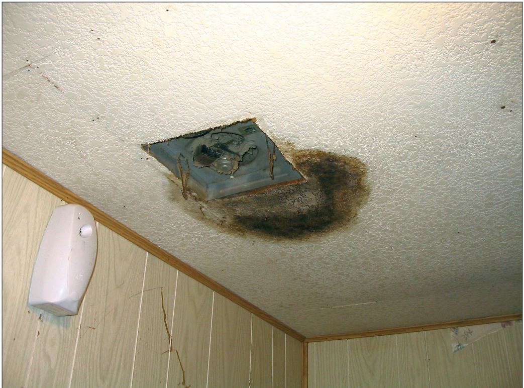
Figure 1. Mould growth around a non-operational ceiling fan.
