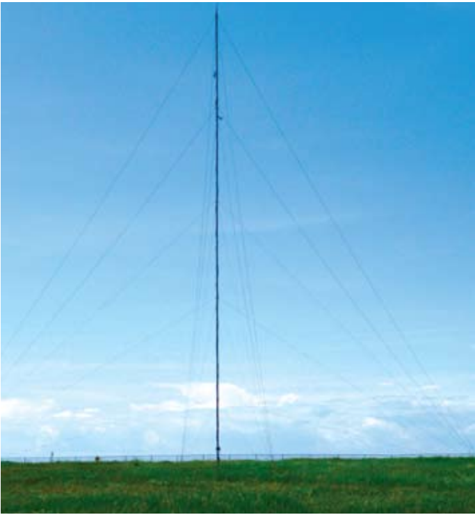
50m wind monitoring tower, Remote Wind Energy Test Site, PEI Photo by: Daniel Van Vliet
