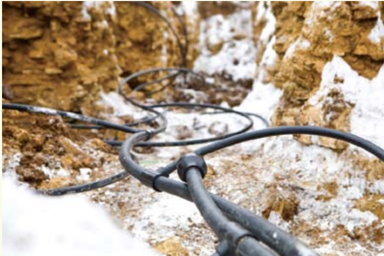
Ground Source Heat Pump Coils
