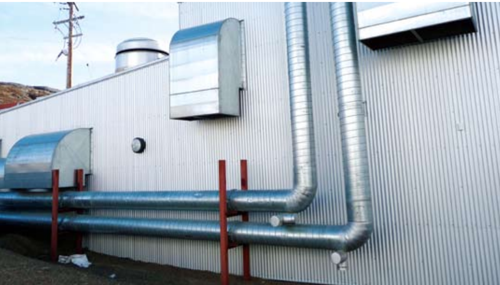
Insulated Pipes Providing Heat to a Community Building in Iqaluit Photo by: Daniel Van Vliet
