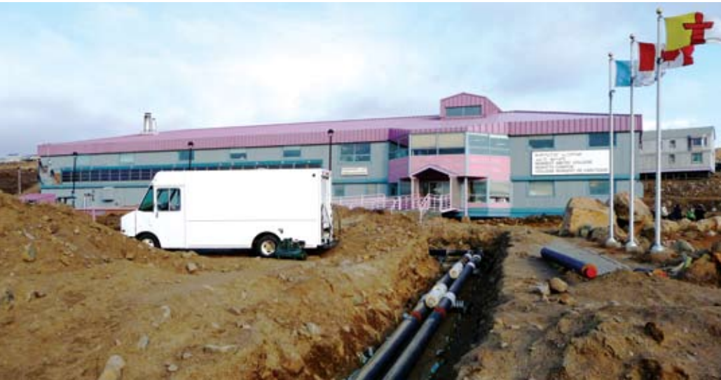
Underground Pipes Carrying Heat from Iqaluit Generating Station Photo by: Daniel Van Vliet
